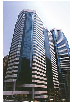
Devon House, Quarry Bay
